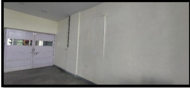
Plate 9: Existing walls of the classroom
