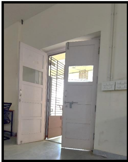
Plate 3: Existing door of the classroom
